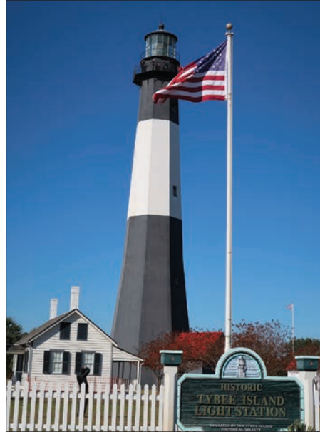
Tybee Island Light Station. Photo courtesy of David Dyjack.
